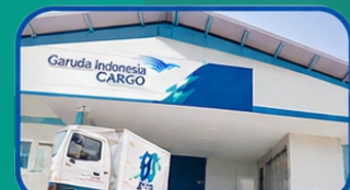
Gedung Garuda Cargo Warehouse
